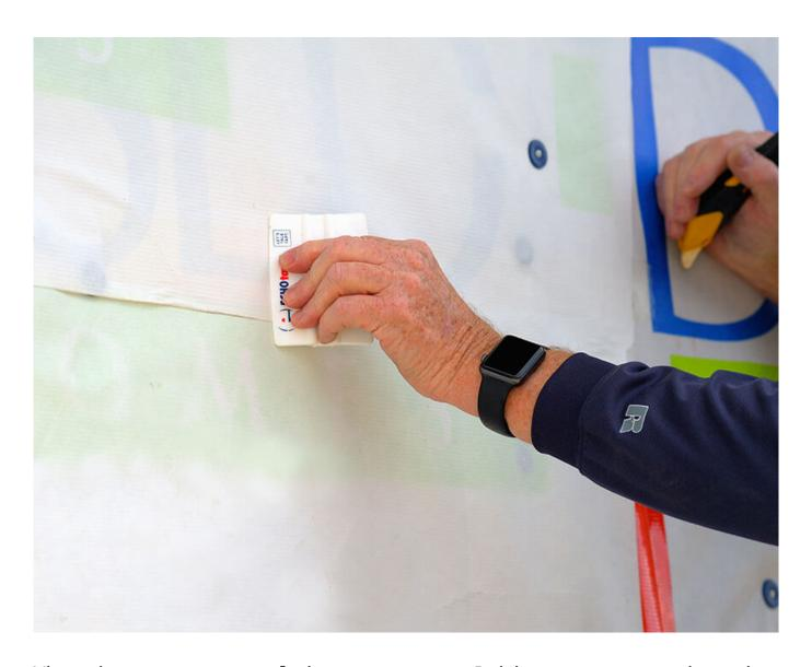
When it comes to applying pressure, Robinson recommends using a squeegee, roller or J-roller in long, even strokes. The appropriate amount of pressure will cause the aggressive adhesive on the seam tape to form a permanent bond with the housewrap within 72 hours.
