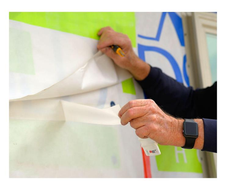
Step 5: Press the housewrap overlap into place using a squeegee or roller.
