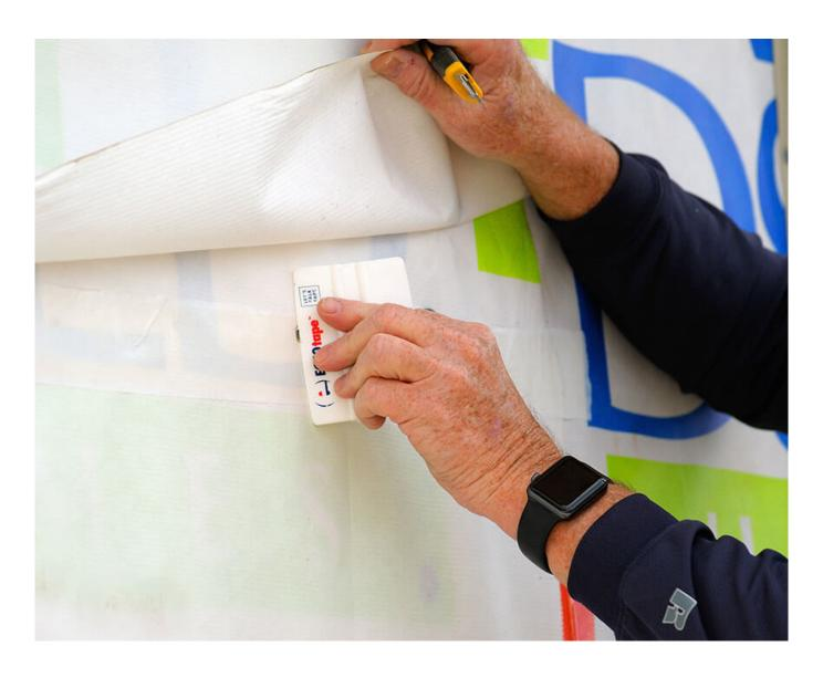
Step 4. Peel back the release liner.
