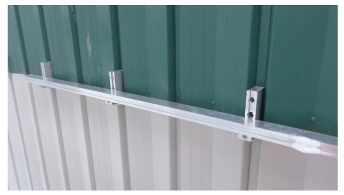
ECHOtape's extreme cold properties allow Green Sun Rising to seal the aluminum profile against the metal façade at the
